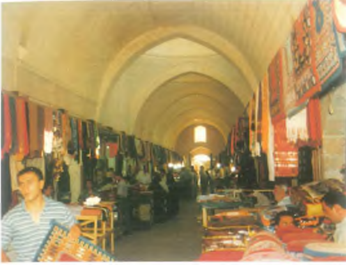
Kazzaz Market Place, after restoration
