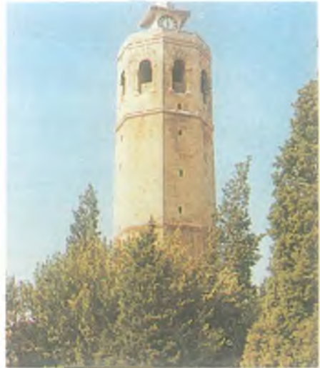
The Minaret of Grand Mosque
