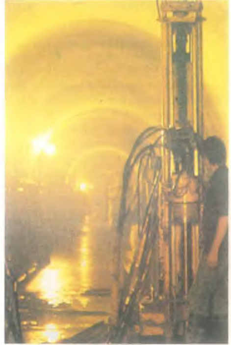
The Urfa Tunnel (Between Atatürk Dam and Urfa)
